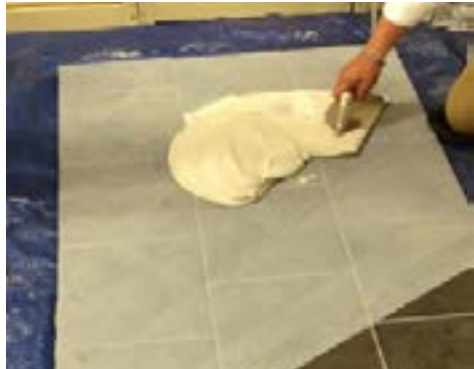
Step 2: Adhesive - applying Mapei UltraFlex LFT thin set
