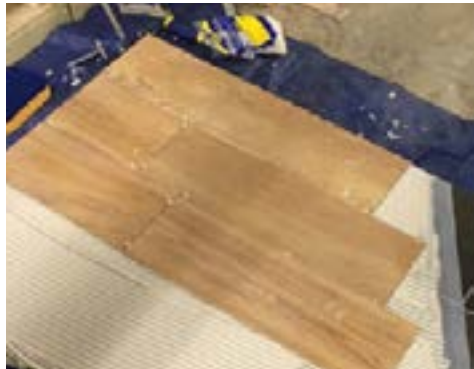
Step 4: Laying tile with spacers & leveling system
