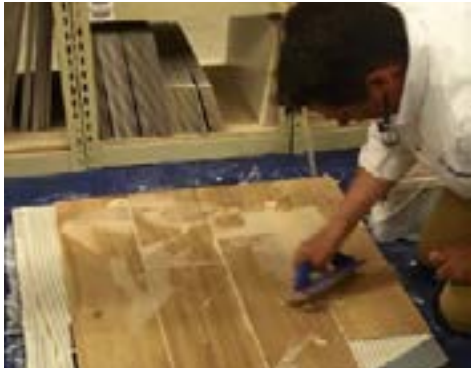
Step 5: Applying Mapei Ultracolor Plus grout
