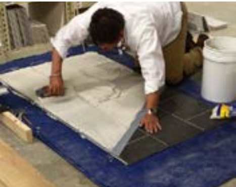
Step 2: Applying thin set with a notched trowel
