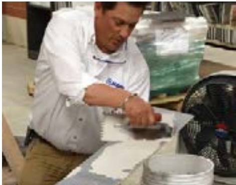
Step 3: Back buttering thin tile
