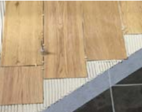
Step 4: Laying tile with spacers
