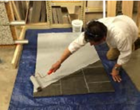
Step 1: Applying Mapei Eco Prim Grip to existing floor
