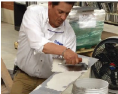
Step 3: Back buttering thin tile
