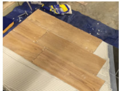
Step 4: Laying tile with spacers & leveling system
