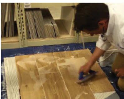
Step 5: Applying Mapei Ultracolor Plus grout
